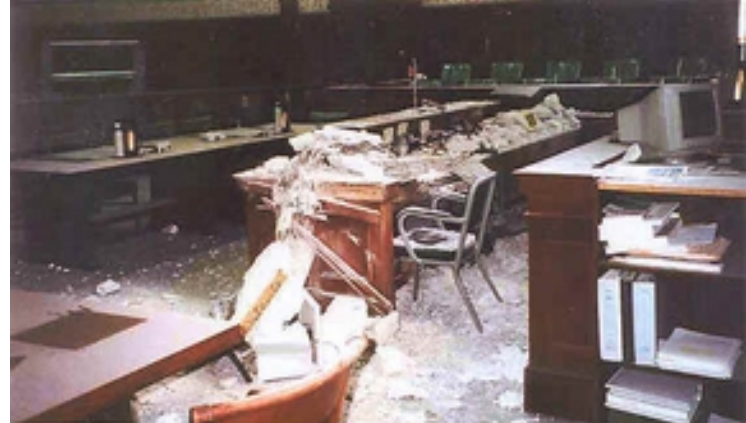
Mercer PA ceiling collapse
